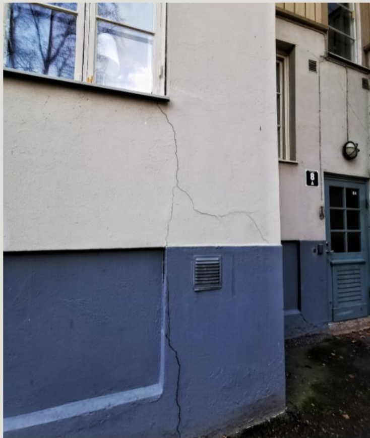
The picture shows a deep wall crack on the building situated between Ågatan and Underåsgatan.
